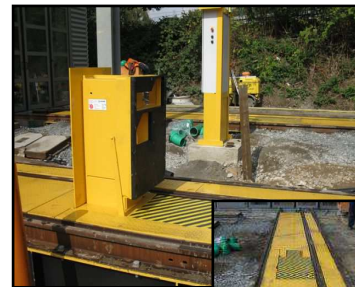
Hinged and cross-over design of the buffer stops and scotch blocks
