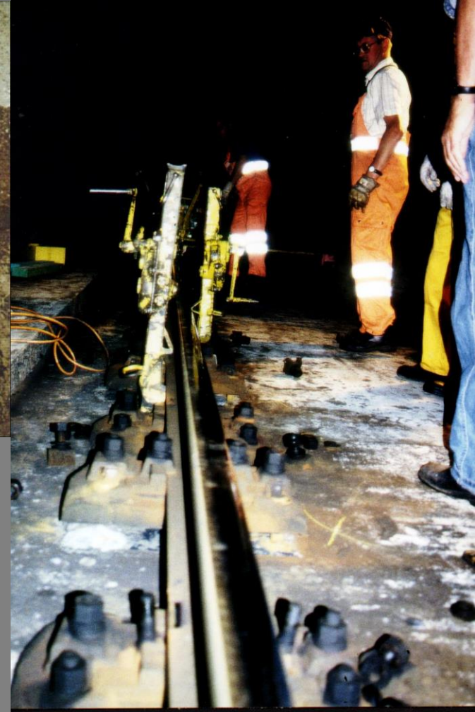
Tearing off by mechanical jacks
